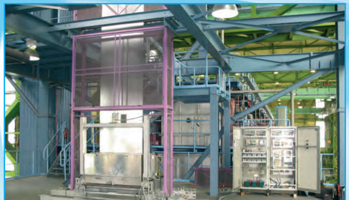
Installation in the cooling section
